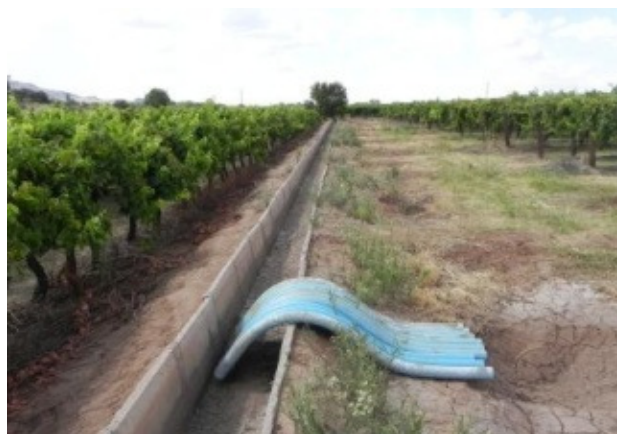
Siphoning system from in-field canal to laser-levelled vineyard flood beds
