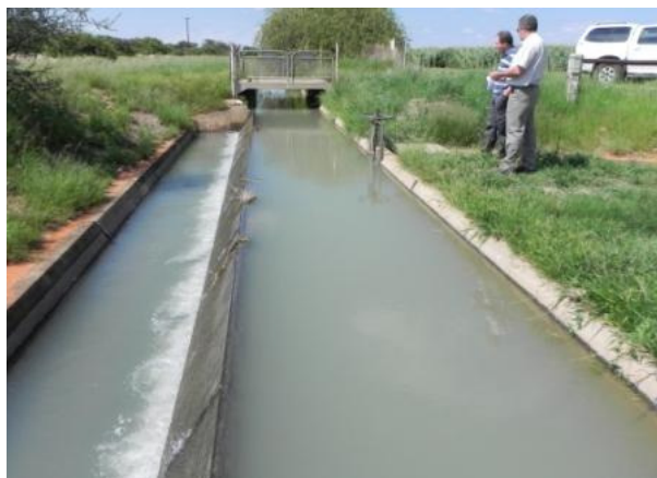
Level-control side weir on Riet canal and distribution sluice gate to Soetmelkvlei Farm
