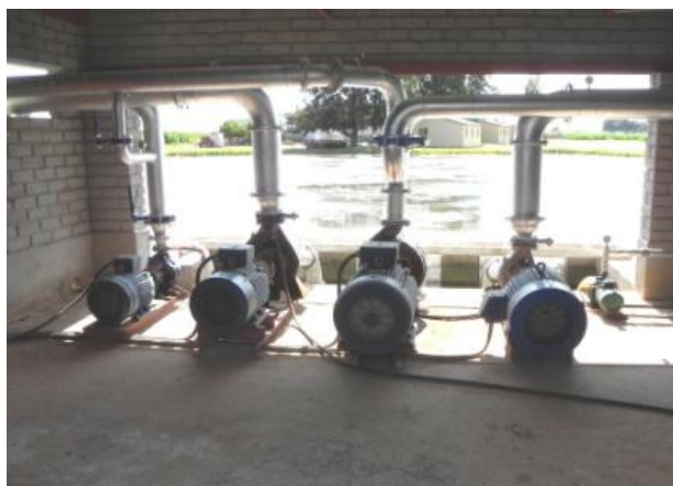
Pump station controlling distribution of irrigation water from storage dam to irrigation areas
