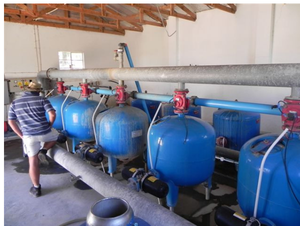
Shelanu farm: Water filtration and "fertigation" system in the pump station
