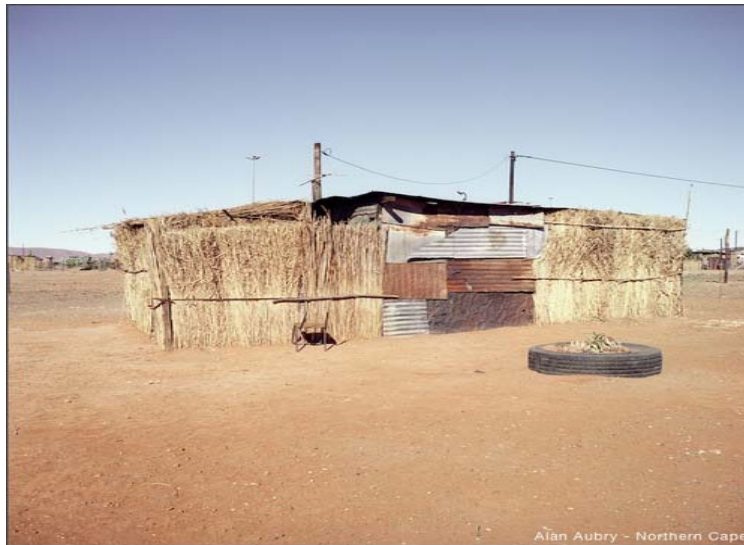
Figure 2: Temporary Structure made from Reeds
