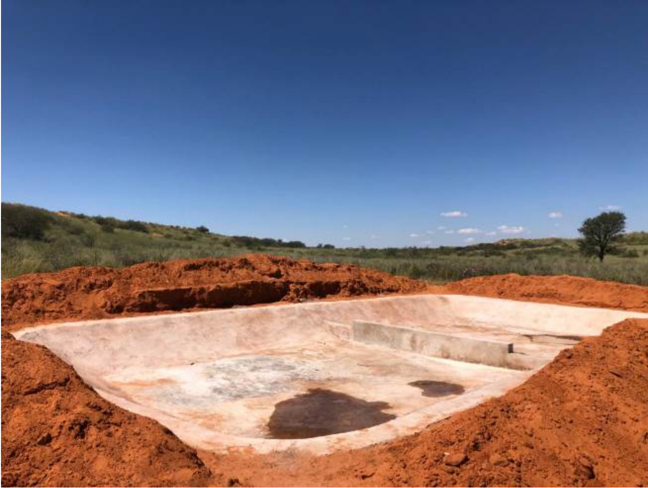
Picture 4: The evaporation pond that serves the desalination plant
